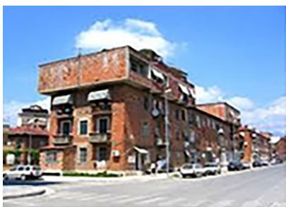
FIGURE 3: Additional unauthorized top of an existing building 14
