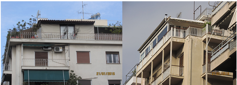
FIGURE 18: Informalities in planned areas that do not exist within the ratified outline of the volume of the building (informal closing of uncovered balconies that are not considered to be within the ratified volume), but can be formalized by Law 4014/2011
