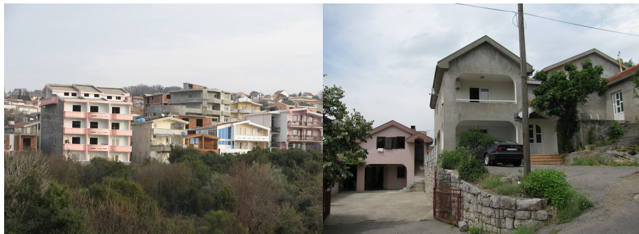
FIGURE 21: Informal development in the coastal area (left) and in Podgorica (right) (photos by C. Potsiou)
