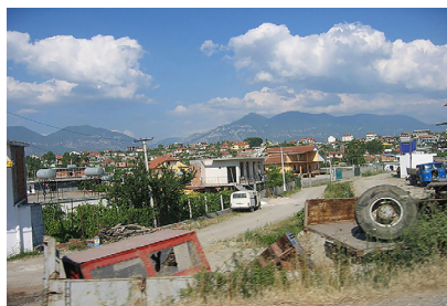
FIGURE 2: Informally build area Bathore in the northern part of Tirana 13
