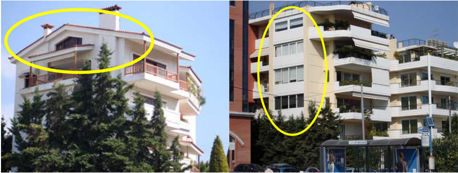
FIGURE 17: Illegal room under the roof of the building (left); Enclosure of semi-open areas that are within the ratified outline of the volume of the building (right) 46
